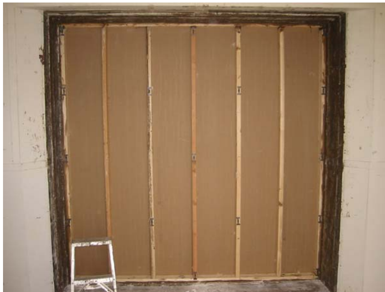
Figure 2: Green Glue® Noiseproofing Clips RC Layout Photo
